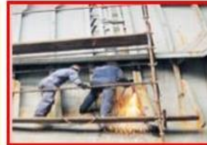
Maintenance/ repair or renewal
